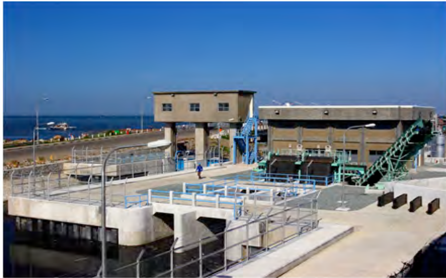
Bangkulasi Pumping Station and Floodgate R-10, Navotas City
