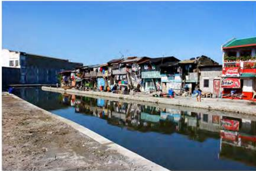
Longos Creek Malabon City
