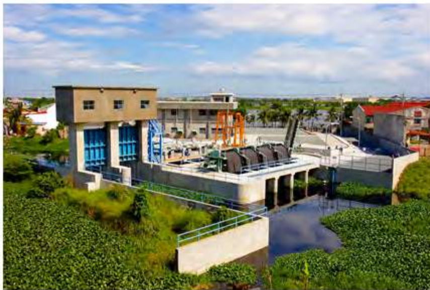
Catmon Pumping Station and Floodgate Gov. Pascual Ave., Malabon City
