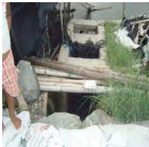
Constructed Tosang within the polder dike
