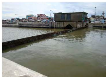
NAVIGATION GATE Tanza, Navotas City (W=25 m, H = 8.9 m)
