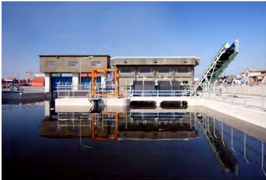
Maypajo Pumping Station and Floodgate Maypajo, Kalookan City
