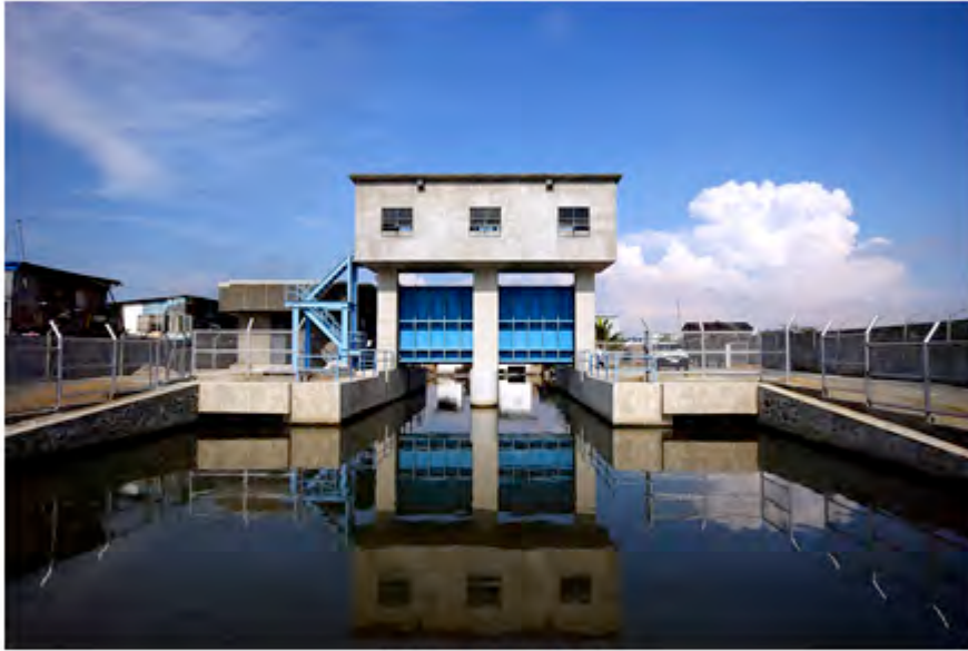
Longos Floodgate Longos, Malabon City (2 x 4.0 m x 4.2 m)
