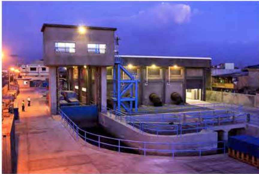
Spine Pumping Station and Floodgate Lapu-Lapu Ave., Navotas City
