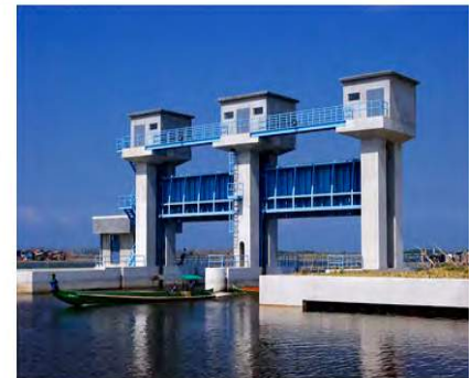
Kallugan Floodgate Dampalit, Malabon City (2 x 12.0 m x 4.4 m)
