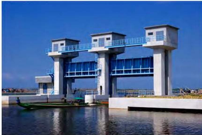
Kailugan Floodgate Dampalit, Malabon City (2 x 12.0 m x 4.4 m)
