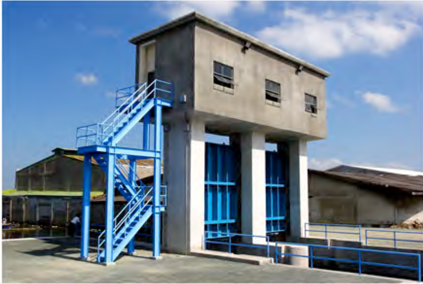
Pinagkabalian Floodgate Dampalit, Malabon City (2 x 4.0 m x 5.4 m)
