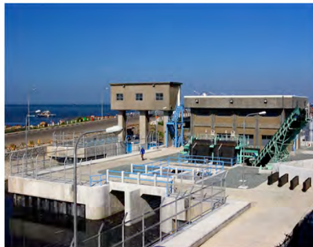
Bangkulasi Pumping Station and Floodgate R-10, Navotas City
