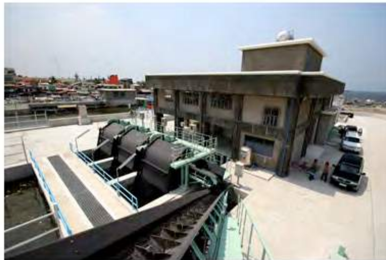
NORTH NAVOTAS PUMPING STATION Tanza, Navotas City
