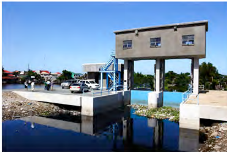
SOUTH PINAGKABALIAN FLOODGATE Malabon City (2 x 4.0 m x 4.0 m)
